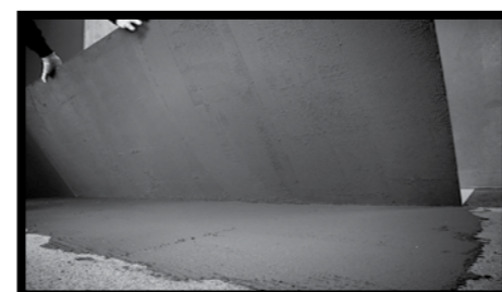
Fig.59 - 2 - Rest the slab on its long side and guide it towards the floor.
