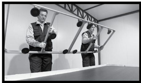
Fig.4/5 - All versions of KERLITE slabs, of size 300x100 cm, can be handled by two persons, using a special frame. Fasten the frame to the slab when it is still on the pallet. Now raise the frame and slab to eliminate the suction effect.
