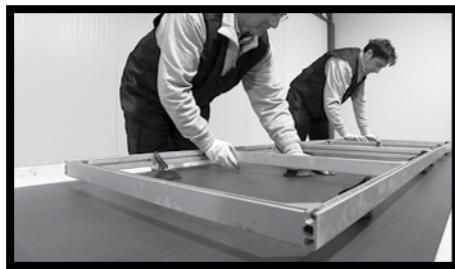
Fig.4/5 - All versions of KERLITE slabs, of size 300x100 cm, can be handled by two persons, using a special frame. Fasten the frame to the slab when it is still on the pallet. Now raise the frame and slab to eliminate the suction effect.
